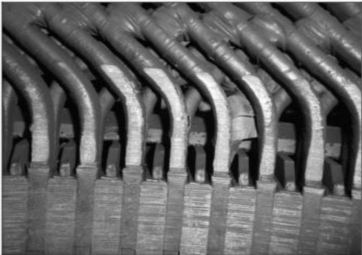
Figure 6 – Stator winding damaged by the bent rods
